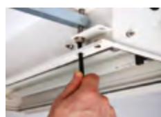
Single screw height adjustment
