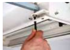
Single screw height adjustment
